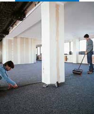
Pressing carpet joint with roller
